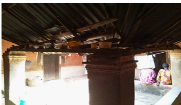
Plate 6(a). Masonry column and roof storage tie-beam Igbara Odo, Ekiti State, Nigeria
