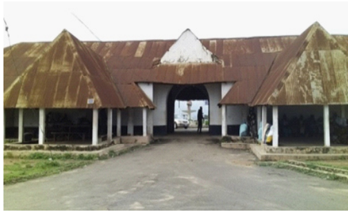
Plate 3(a). Comparing high slope royal gabled roofs of old Oyo palace
